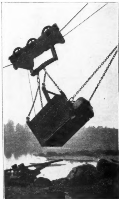
Bucket Used in Digging Gravel
